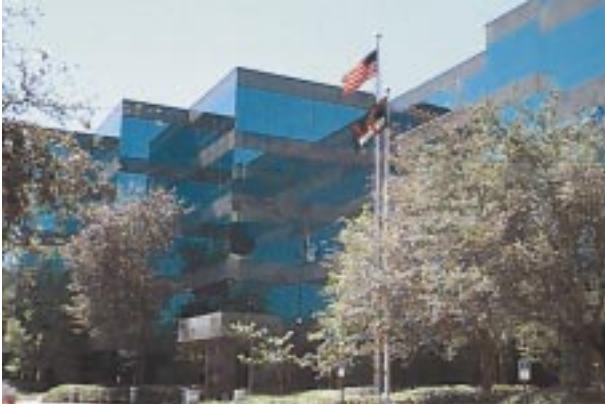
Verizon Data Services Riverside Building Temple Terrace, Florida
