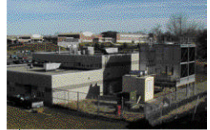
South Campus Chiller Plant ▼
